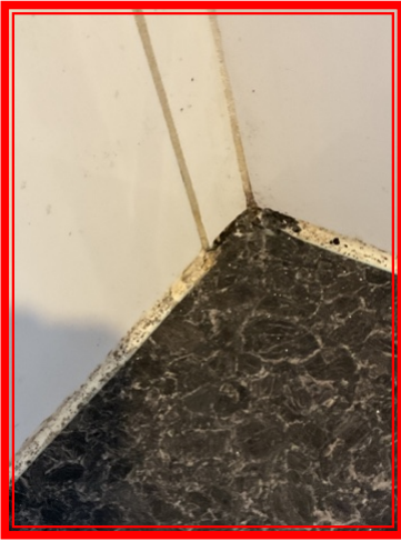
3.13.1 KITCHEN/ WORKTOP(S)/ WORKTOP(S) Mould to mastic around edges .
