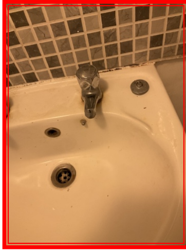
4.10.1 BATHROOM/ BASIN/ BASIN Stains and mould visible .
