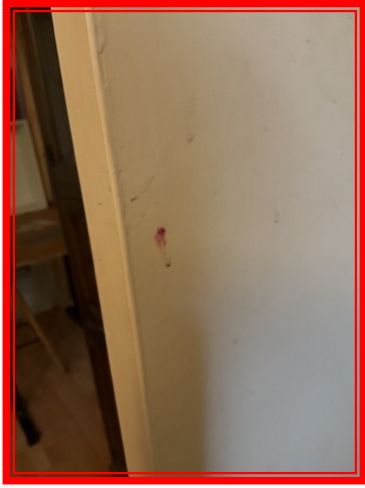
5.1.1 Marks visible to both sides of door .
