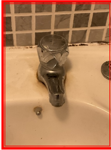
4.10.1 BATHROOM/ BASIN/ BASIN Stains and mould visible .
