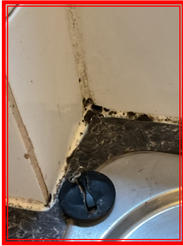
3.13.1 KITCHEN/ WORKTOP(S)/ WORKTOP(S) Mould to mastic around edges .
