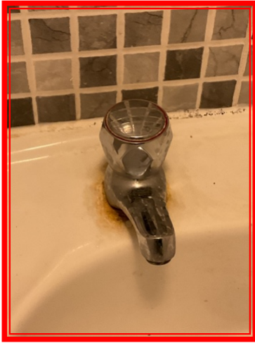
4.10.1 BATHROOM/ BASIN/ BASIN Stains and mould visible .
