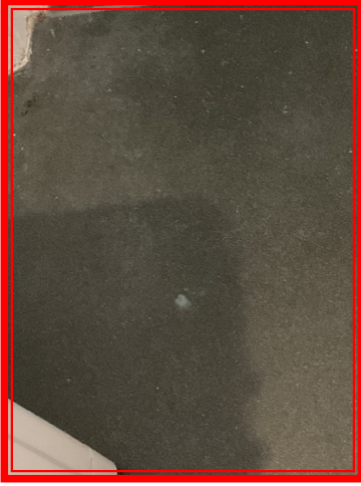
3.13.1 KITCHEN/ WORKTOP(S)/ WORKTOP(S) Mould to mastic around edges .
