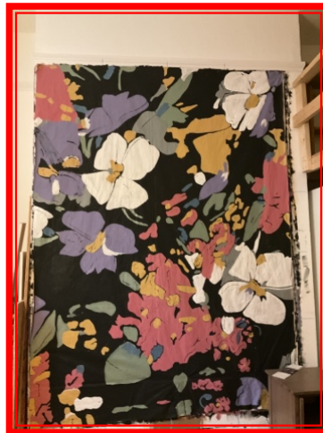
5.4.1 Large painting fitted, with multiple paint marks to wall below .
