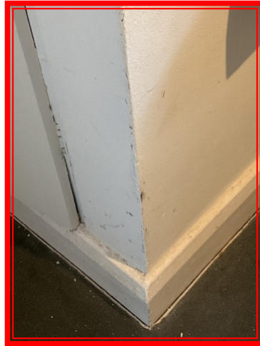
3.5.1 KITCHEN/ WALL/ WALL Marks and signs of wear to lower sections visible .
