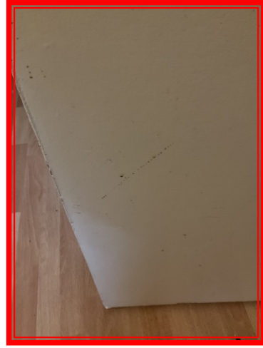
5.1.1 Marks visible to both sides of door .
