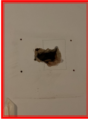
5.4.1 LOUNGE/ WALL/ WALL Damage to walls throughout, large hole to RHS of windows .
